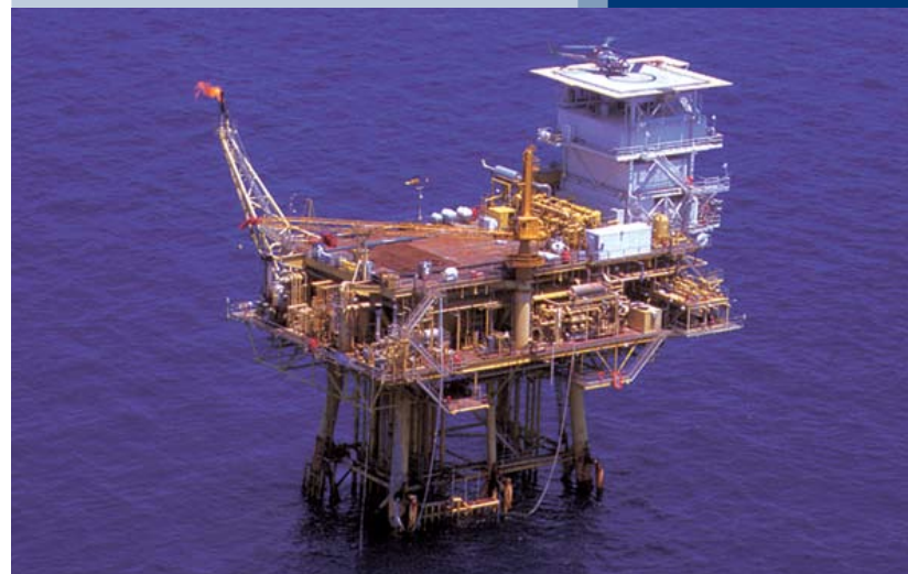
High Island A389A Production Platform, FGBNMS
